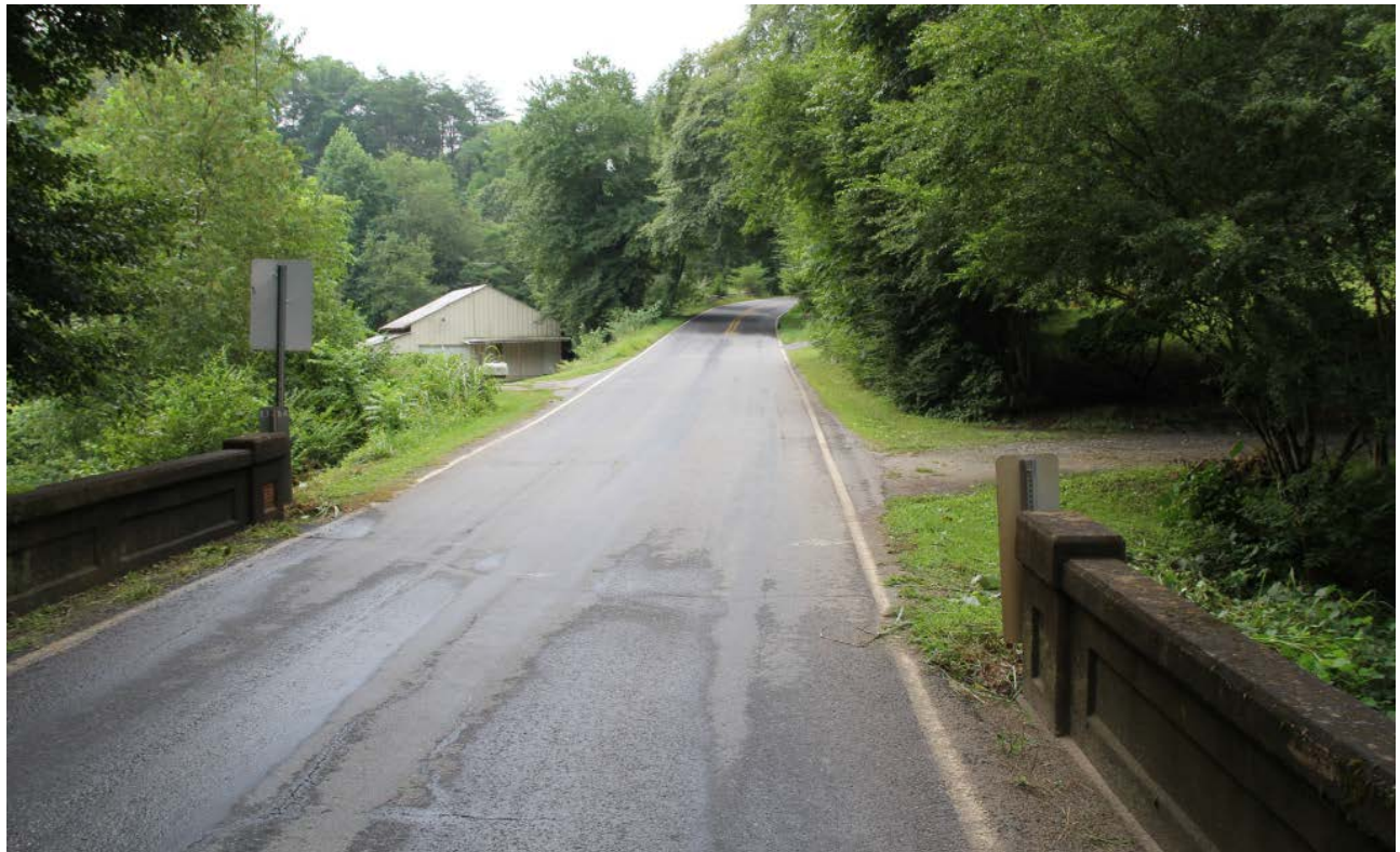
View south along SR 1140 (Myers Chapel Road) from Bridge No. 87
