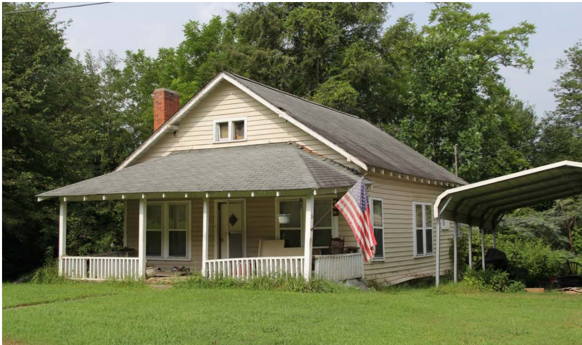
House, 2910 Myers Chapel Road, view to west
