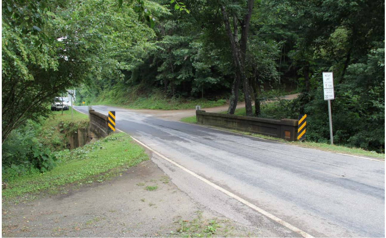
Bridge No. 87 on SR 1140 over Hyatt Mill Creek, view to northeast from West House driveway
