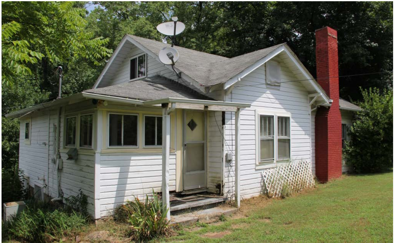
West House, oblique rear view to northeast
