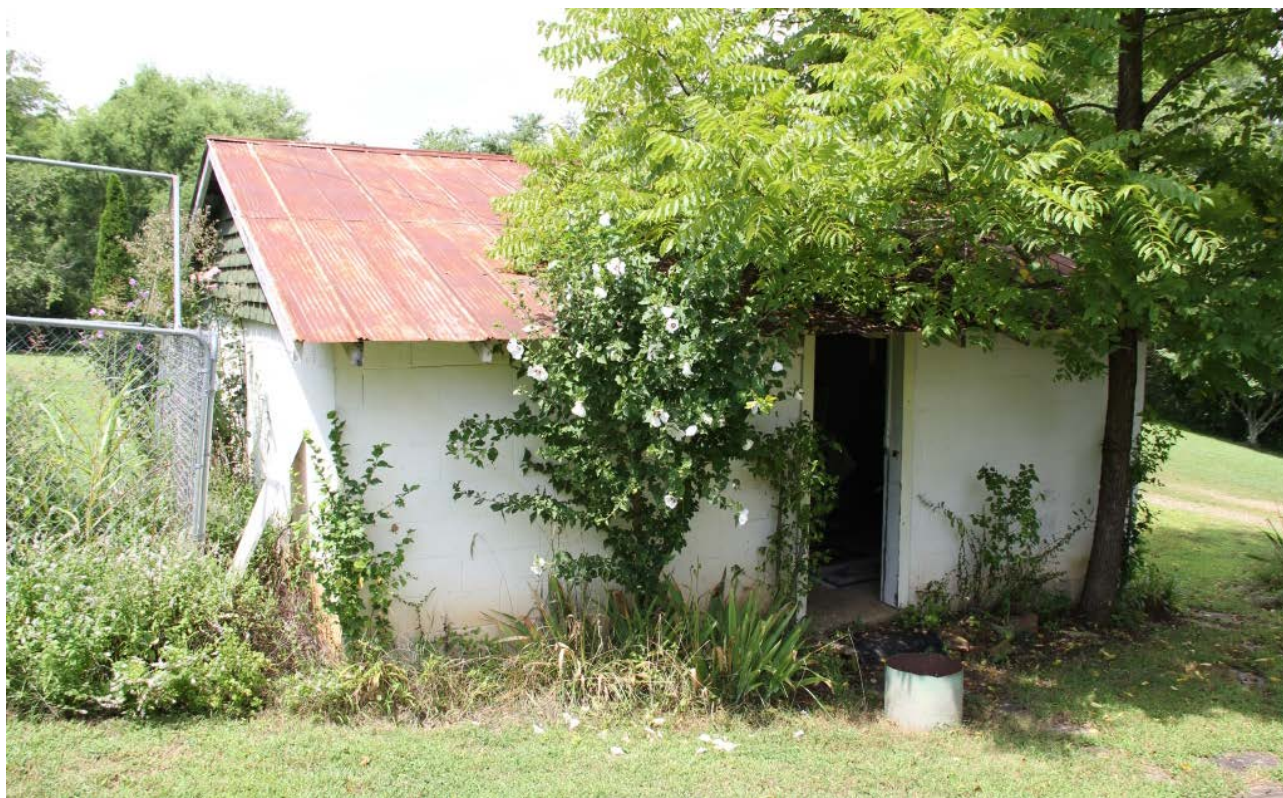
Garage, east elevation, view to northwest
