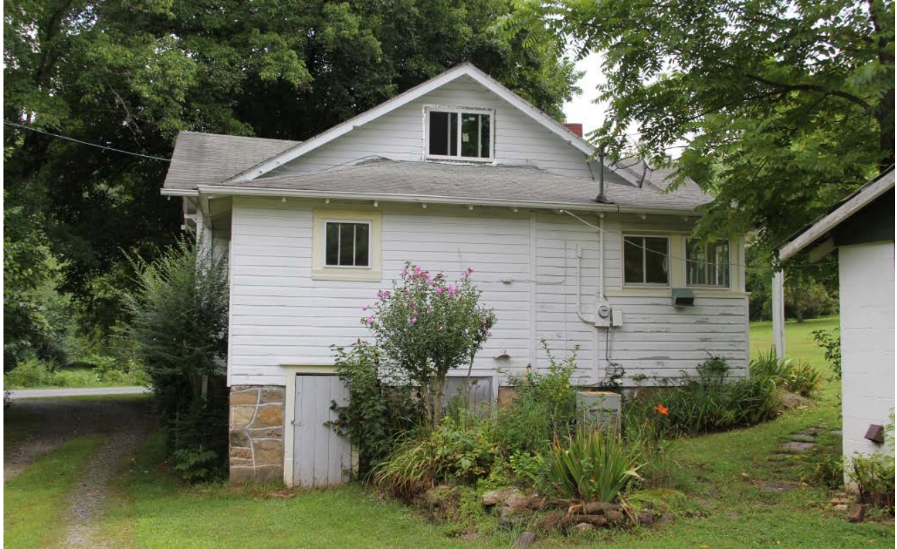
West House, rear elevation, view to east
