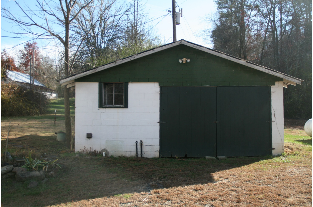
Garage, façade, view to south
