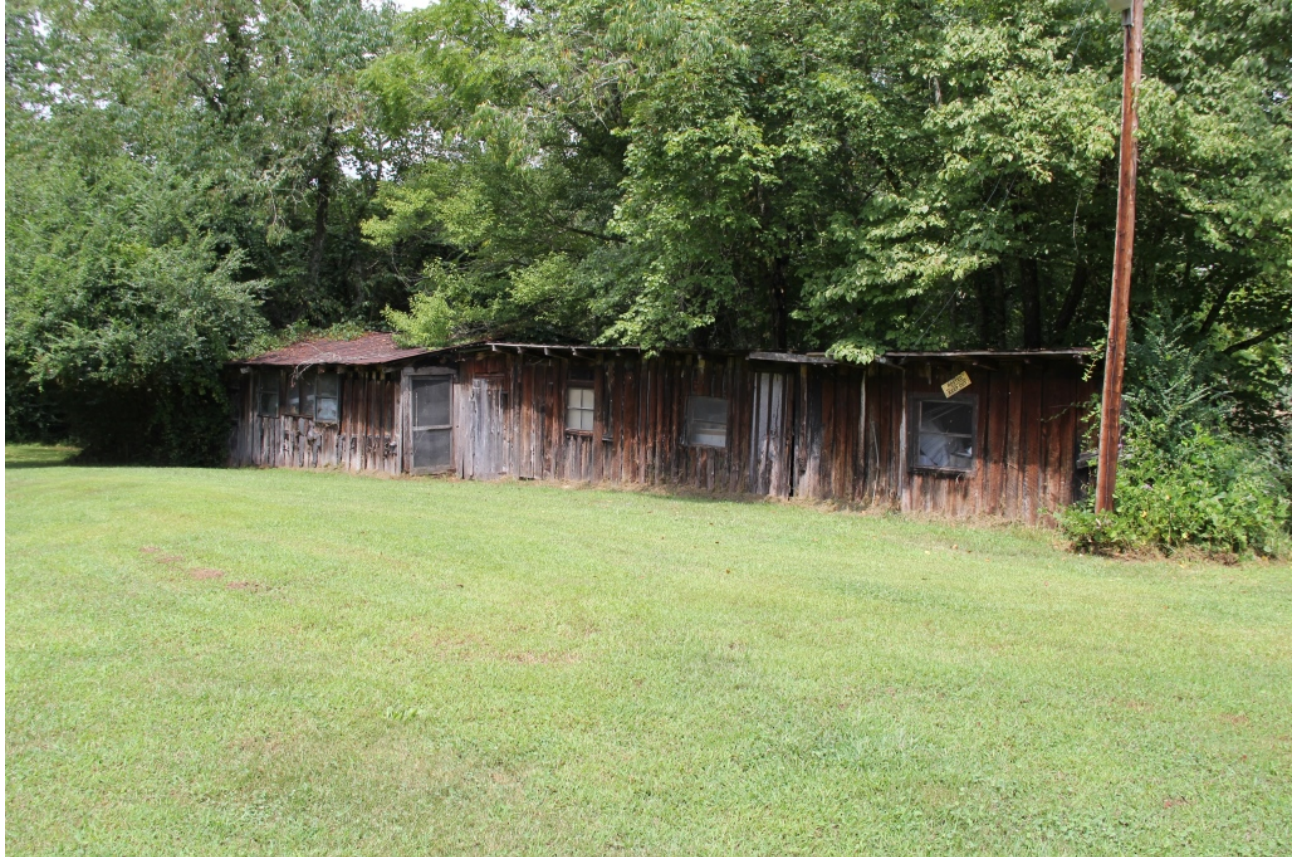
Chicken coop, oblique front view to northwest
