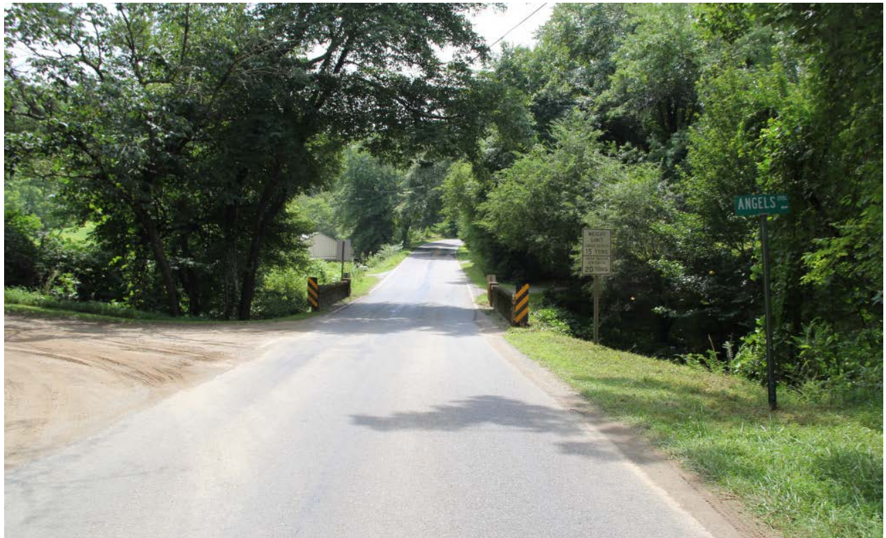
Bridge No. 87 on SR 1140 (Myers Chapel Road), view to south
