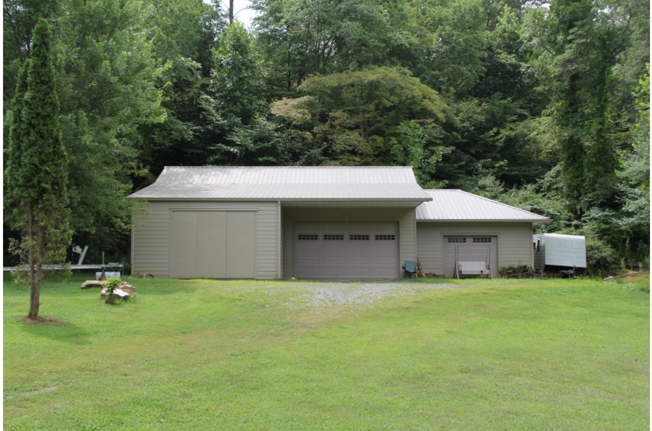
Workshop, façade, view to southwest
